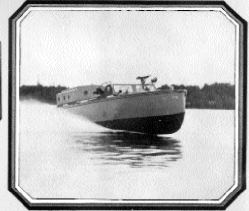
"Canadian Customs Patrol Boat "BEHAVE," one of a fleet of six developed for duty on the rough waters of the Atlantic Coast. Armed with machine guns and with full load and equipment these boats travel at 33 m.p.h. with 300 h.p.
